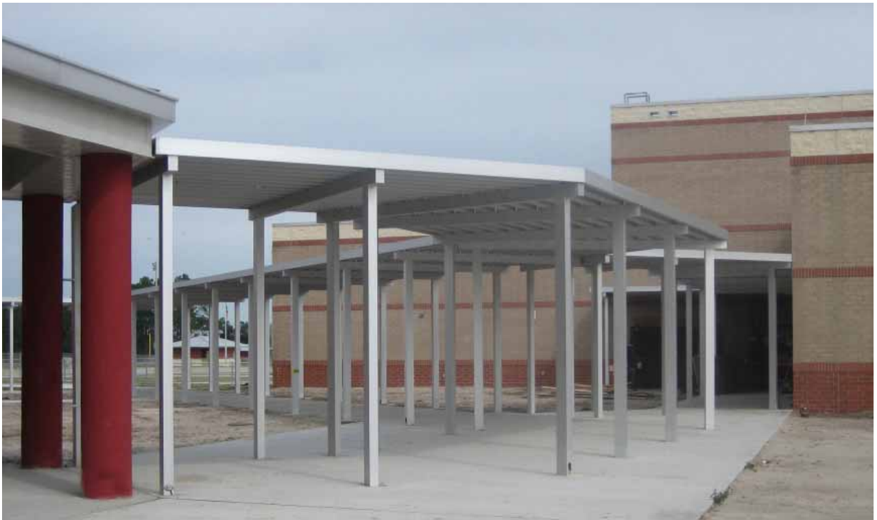
T. DEWITT TAYLOR Pierson, FL H.J. High, Contractors
