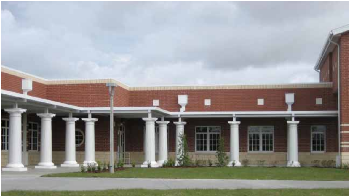
LIBERTY HIGH SCHOOL Ocala, FL M.D. Building Systems, Contractors
