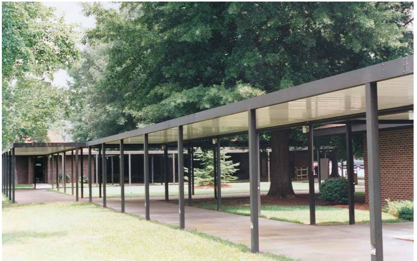
NASH GENERAL HOSPITAL Rocky Mt., NC Flora's Glass, Contractors
