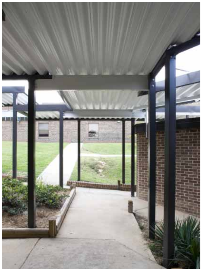
BEVILL STATE COMMUNITY COLLEGE Sumiton, AL Creative Aluminum, Contractors
